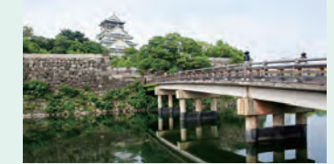
K Gokurakubashi Bridge
